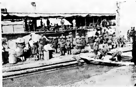
LANDING STORES AT ARAB VILLAGE.
